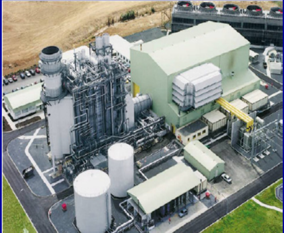
2 X 350 MW CCGT under construction
